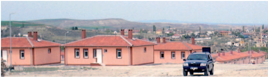
Figure 4 | The new village of Tuzkoy. The new village is built with bricks and cement; the old village can be seen in the background. The new village should open in the summer of 2007 or as soon as the roads are covered with asphalt and the sanitation system is completed.
