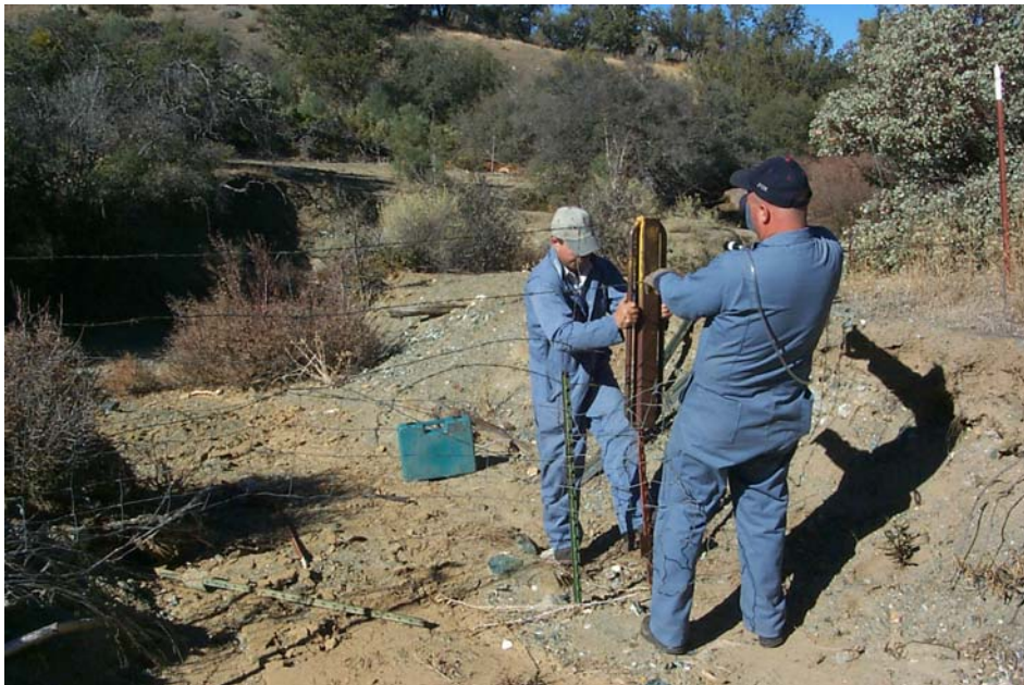
BLM implementation personnel repairing a fence along sensitive species habitat
