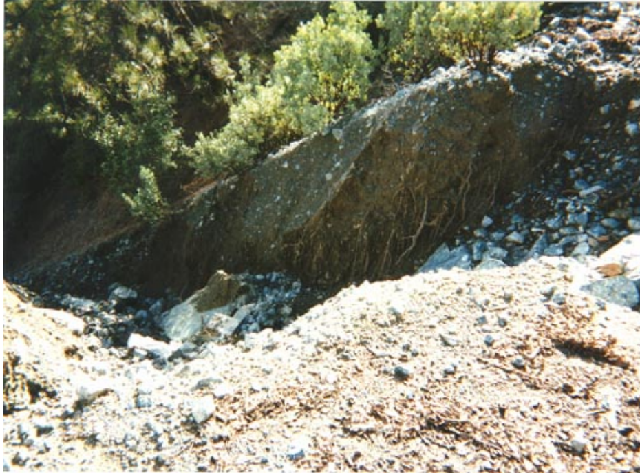
Erosion along a route
