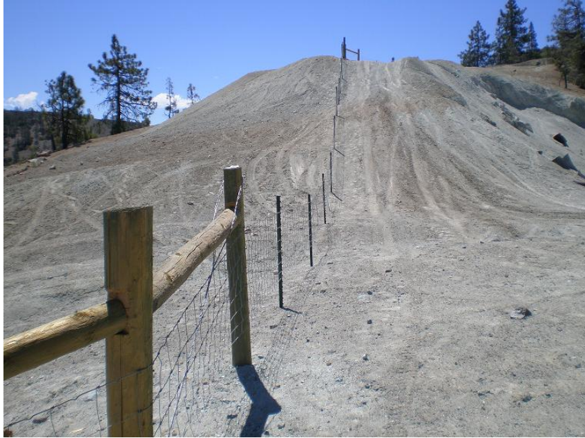
Photo 2. New fencing along R14 to prevent OHV entry to closed area (Aurora Mine) and the SBMRNA.
