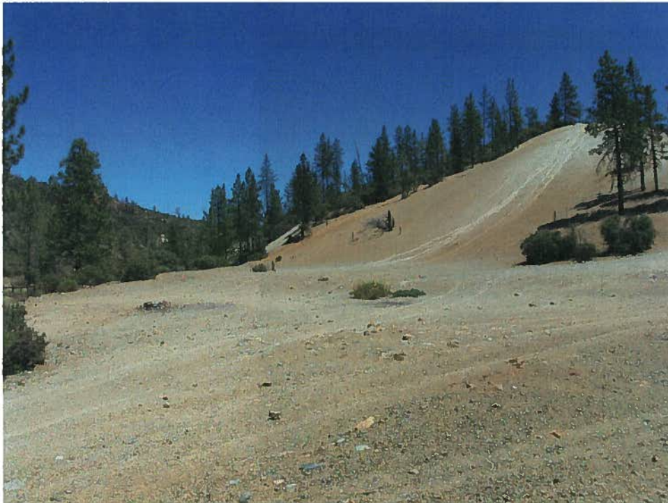
Figure 7. SA 4 (Indian Hill). Sediment averaging 6 inches deep covers most of the SA. Soils are compacted. Most of the sediment originated from the large barren hillclimb slope in the background.
