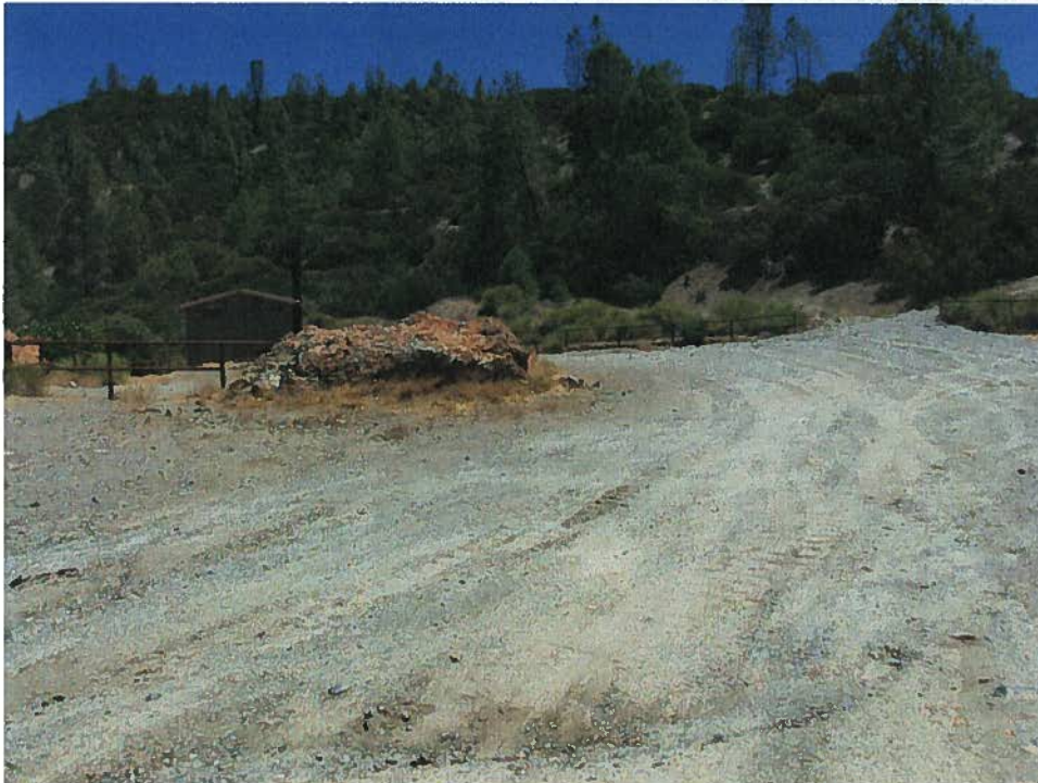
Figure 5. SA 2. Sediment averaging 7 inches deep covers most of the SA. Soils are compacted. Most of the sediment originated from T108 which departs from the SA up the slope in the background.
