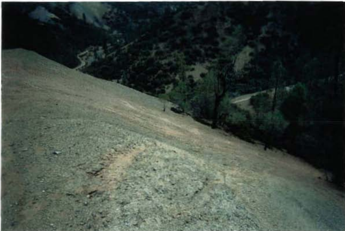
13) Looking NW from CL-24. Well armored steep inner gorge leading to Clear Creek.
