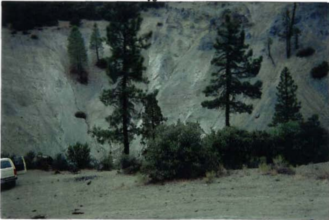
22) Looking NE from the bottom of CL-30. Evidence of mass wasting due to slides.
